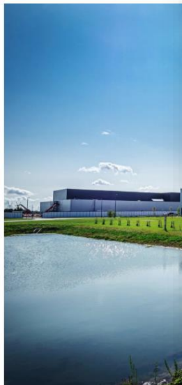
Facebook Data Center in Odense, Denmark
